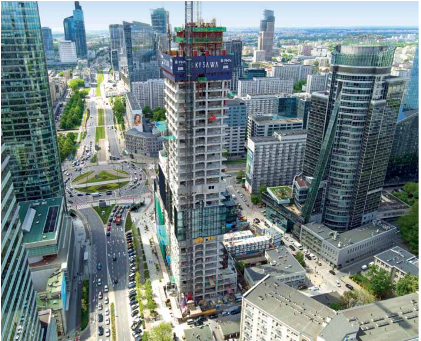
Multiple records for one tower: The 155-metre SKYSAWA pencil tower dominates the Warsaw skyline with 40 floors and a total area of 40,000m 2 . Built by PORR, which is once again setting records with future-proof technologies and a pioneering spirit.
