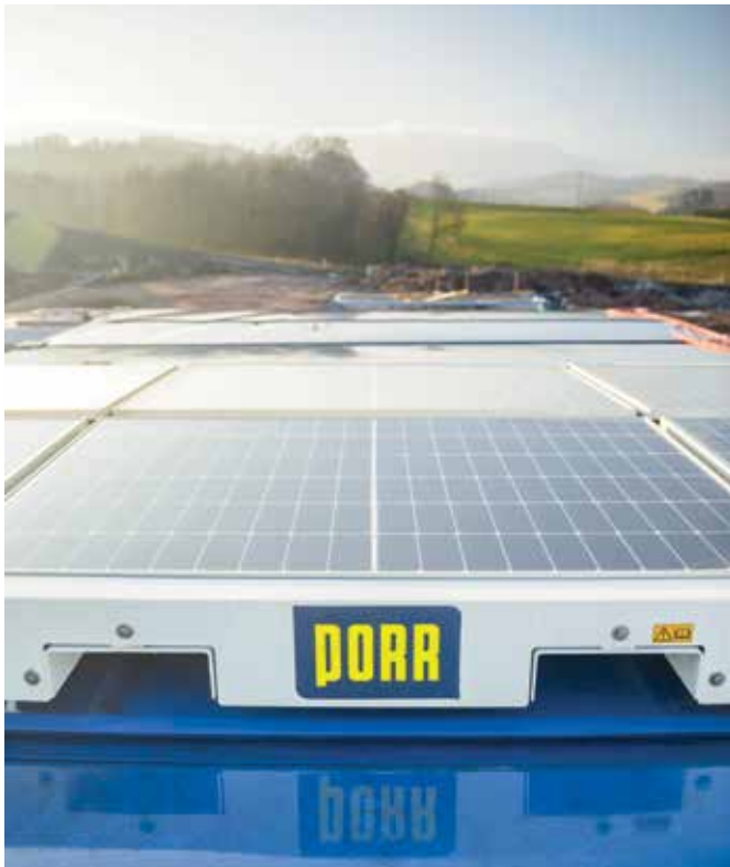
The mobile solar panels on the S3 motorway project in Poland work on the plug-and-play principle and can be put into operation easily and quickly.
