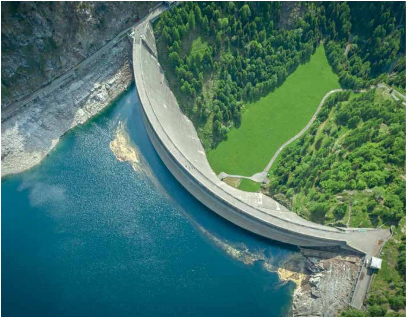
At the Mooserboden storage power plant in Kaprun, an intake and outlet structure separates the two existing dams at around 2,000 metres above sea level. The main challenge of this project was the large number of workstations, some of which were located in the high alpine region.
