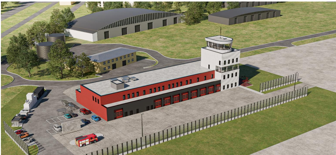
PORR is delivering the first construction phase of the Aerial Port of Debarkation (APOD) at Wrocław-Strachowice Airport © RZI
