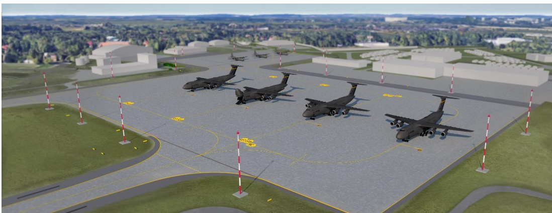
Construction works on APOD will continue to 2029 © RZI
